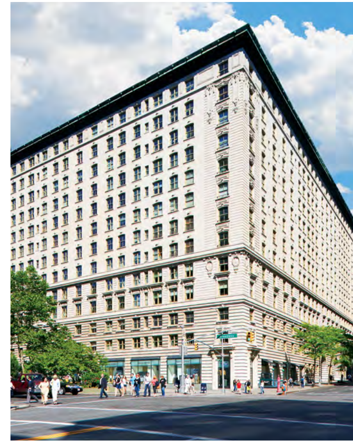
Upper West Side
